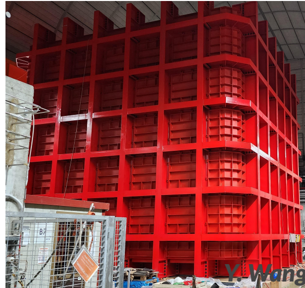
DarkSide-20k: Under construction at LNGS
